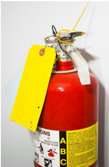
Figure 5 - Fire Extinguisher with Inspection Log.
