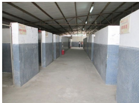
Figure 29 - Best Practice Hazardous Waste Storage Segregation
