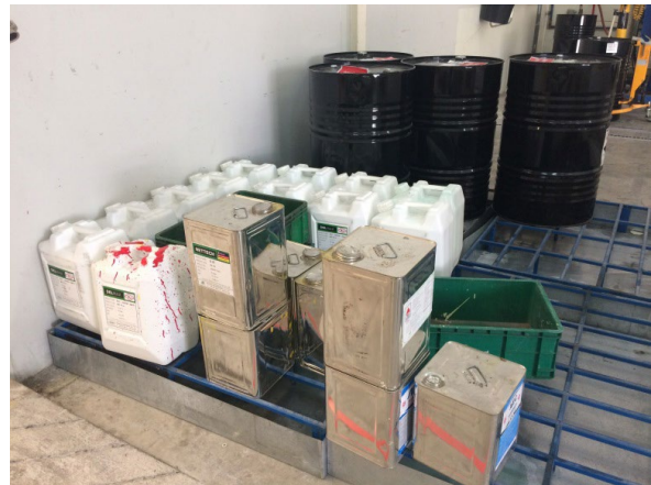
Figure 19 - Chemical Storage Room with Secondary containment device.
