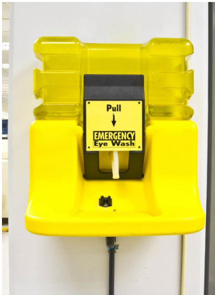
Figure 18 - Eye Wash Station
